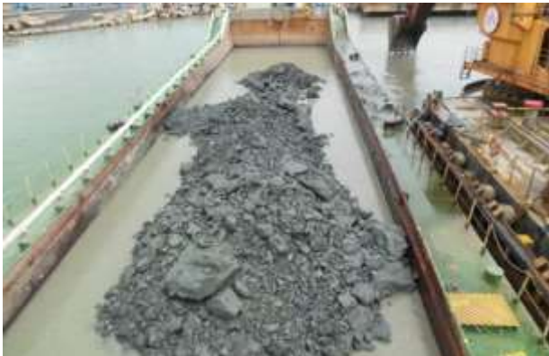
Figure 5.1-1 Rock dredged by backhoe dredgers
